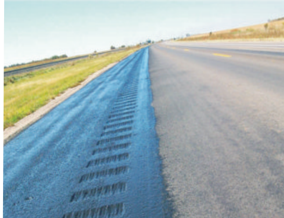
Shoulder Seal over Rumble Strips
