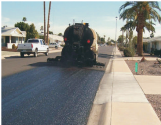
Modified Surface Sealing- Residential Open Grade
