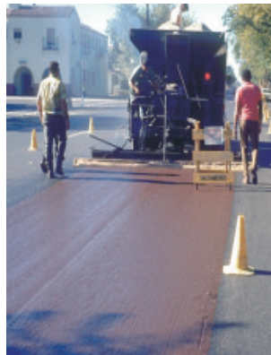
Slurry Seal is Placed
