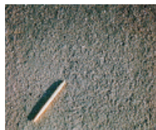
Chip Seal is Paced
