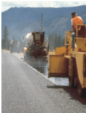
Chip Seal is Paced
